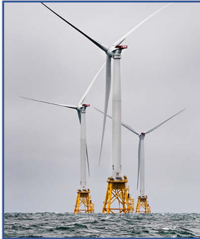
Figure 37. Offshore Wind Turbines Source: Dennis Schroeder | NREL 40484
